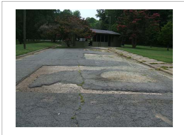
The Tennis Court Parking Lot (not slated for repair or renovation)
